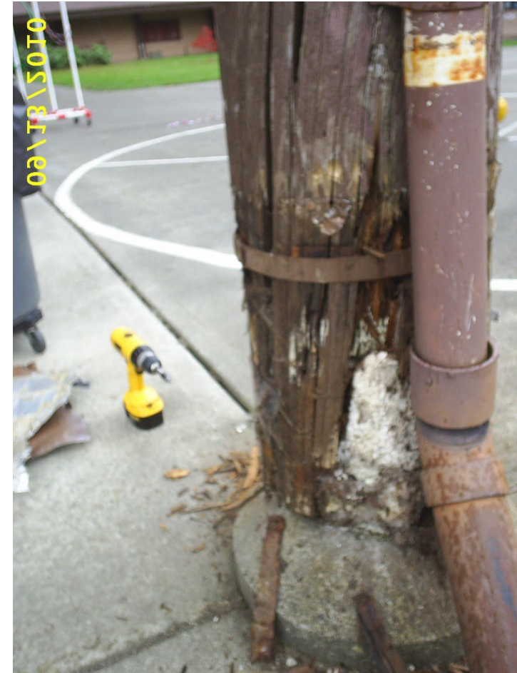
Monroe – Emergency Repair Pool – Beam Replacement..
